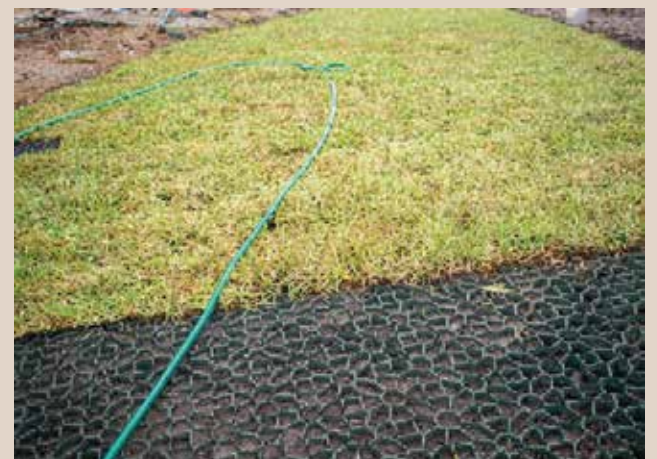
Path on established lawn with D-Smart Flooring
