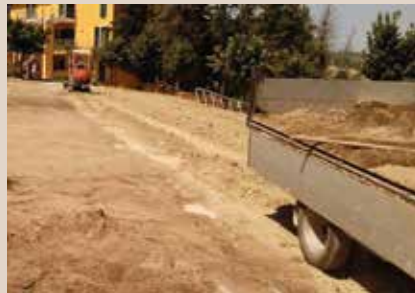
Preparation of foundation layer
