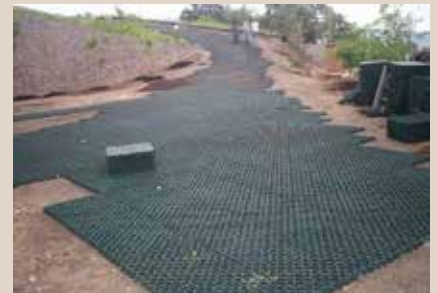
Lay the Decoland Smart Flooring
