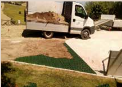
Filling the cells with organic soil
