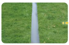
Uncoil the B-Edge Pro (XL) by putting a weight at the ends during mild ambient temperature, preferably in the sun. This allows the edge to flatten.
