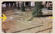
Extend individual L-Edges using the connector by insertion into the holes provided for. After final positioning of the edges, use the galvanized steel anchors to fix the position of the edges, install 2 anchors for every 100 cm.
