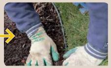
Whilst keeping the edge down, push firmly the soil against the D-Edge Smart Pro to fix it.
