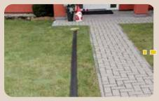
Uncoil the D-Edge Smart Pro by putting a weight at the ends during mild ambient temperature.
