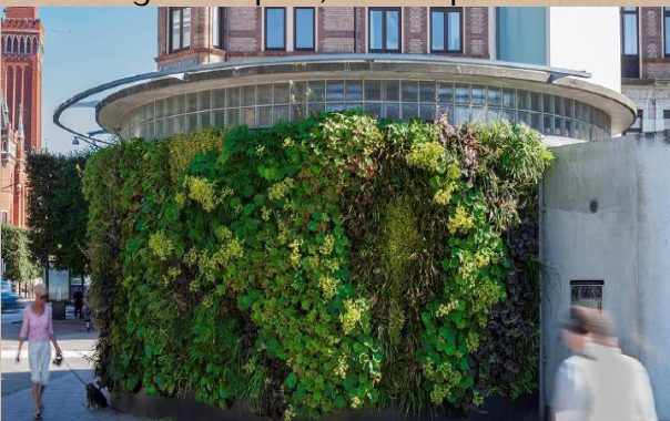
Pump house, Helsingborg - Sweden
